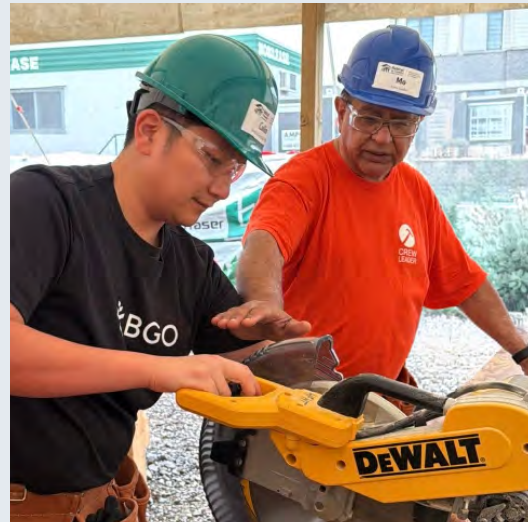
Habitat for Humanity Build Day in Brampton, Ontario, Canada
